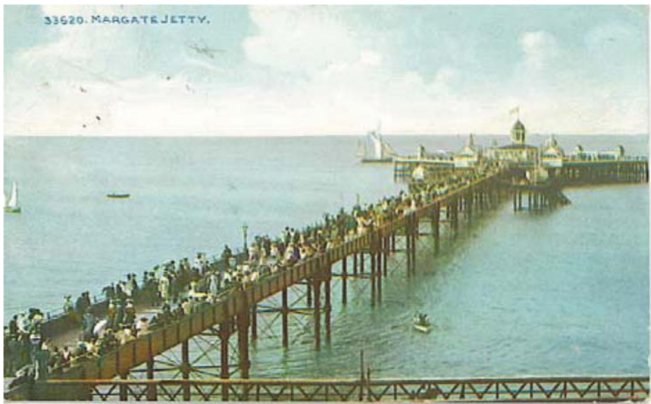
FIGURE 6 Period postcard of Margate Jetty built on screw-piles (Author's collection).
